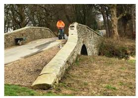
**Figure 20** The bridge, prior to restoration work, showing unstable coping stones *Quarry Investments Ltd*.
