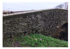
**Figure 22** The bridge, prior to restoration work, showing missing rubble stones at the base of the bridge *Quarry Investments Ltd*.
